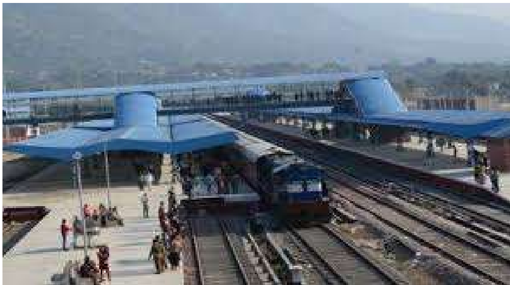
Fig 12.9: Kathgodam Railway Station, Source: Google
