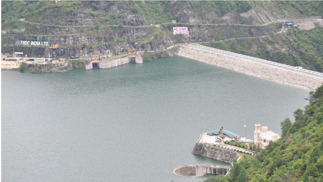
Fig 11.9: Teri Dam, Source, Google
