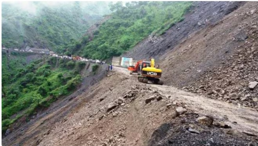
Fig 13.2: Landslide, Source: Google
