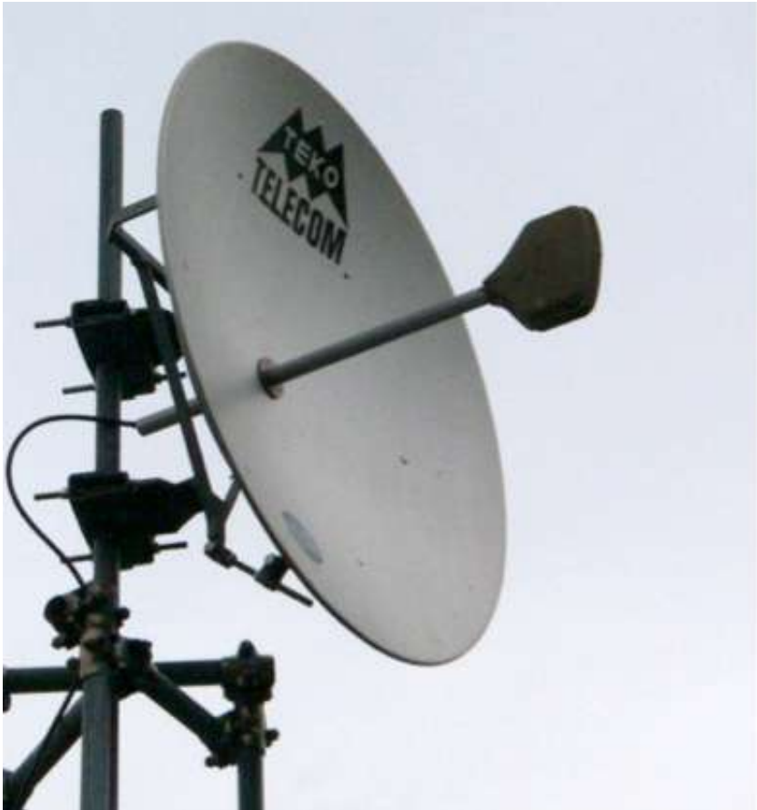
Figure ATL 14: A solid dish antenna.
