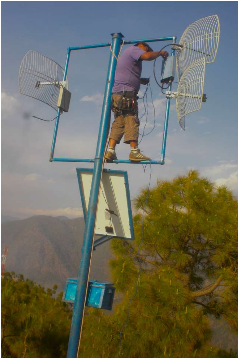
Figure CSD 8: Backhaul Relay, Garhwal Network
