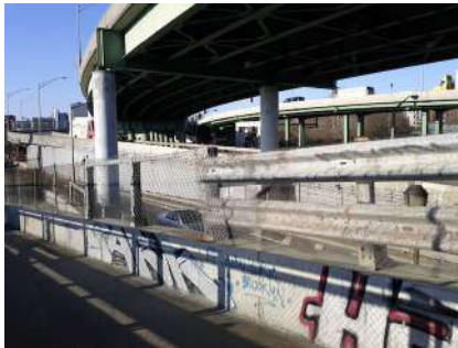
Figure CsOTI 3: Gowanus Expressway which divides the Red Hook neighborhood from the rest of Brooklyn.
