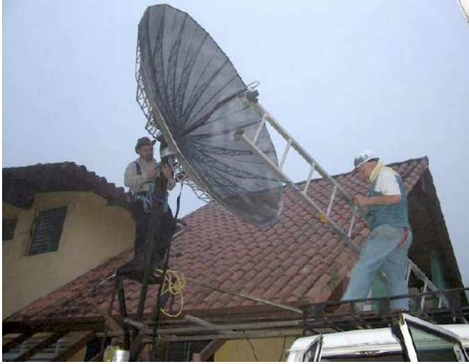
Figure CsLD 5: Carlo and Ermanno disassembling the satellite dish supplied by Mr. Ismael Santos.
